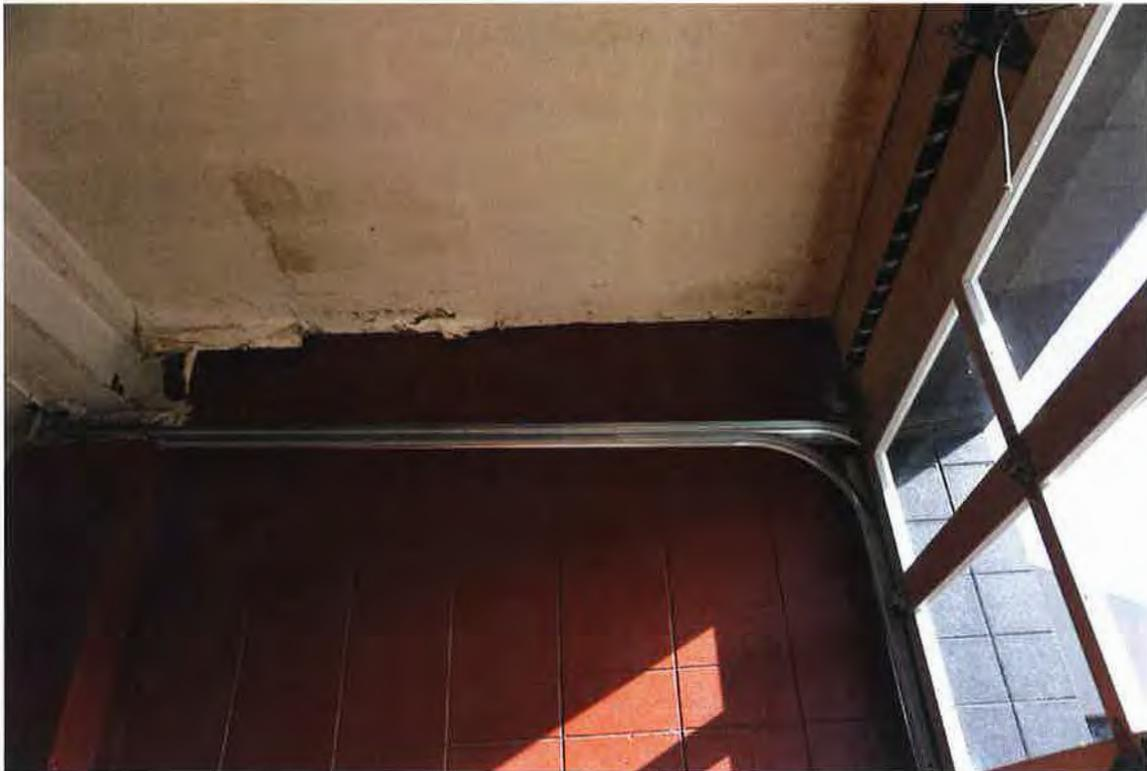
Leaking Roof Ceiling on North Side of Station 50
